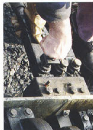
Fig. 1a): Plunger measurement: plunger location (a white element on the point rod, between the point machine and rail)
