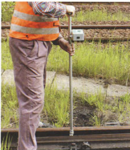
Fig. 5a): Measurement of setting forces using a direct method: measurement with an instrument
