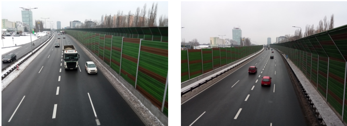
Fig. 3. Using highway noise barriers on the A4 motorway in Katowice
